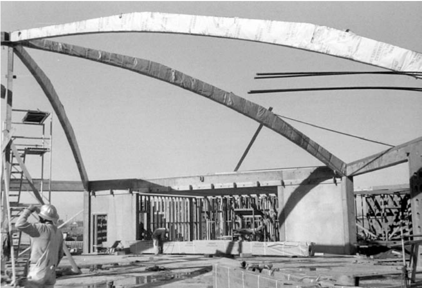
Installing the laminated wood arches at Sierra Boulevard Site
