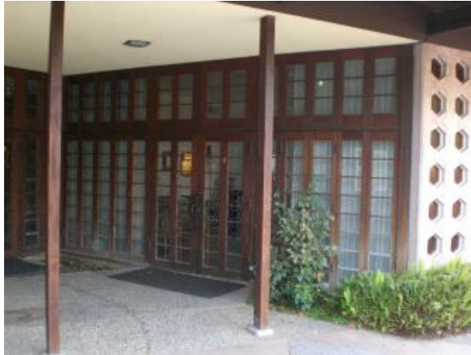
Figure 20- Typical window wall extending to ceiling.
