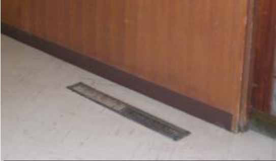
Figure 9- Perimeter heating vents.
