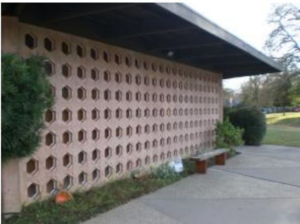
Figure 5 – Concrete tilt-up wall with window perforations.
