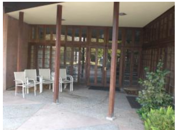
Figure 6 - Window walls with glass doors.
